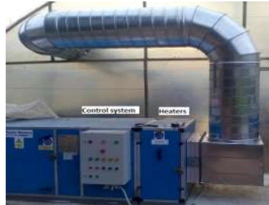
Figure 4: The auxiliary heaters and the dryer control system
