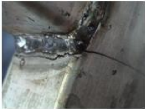
Figure 10: Crack resulting from the fatigue testing, left side of the specimen test
