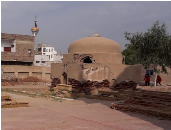
Figure 3: Deteriorated condition of Mir's Tomb site, Source: Author
