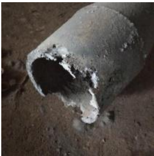
Figure 1: Example of Porous Defect
