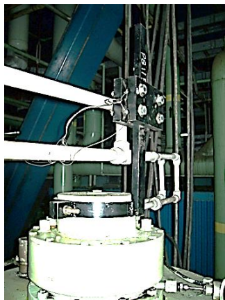
Figure 4: Installation of Vibration Absorber on CEP
