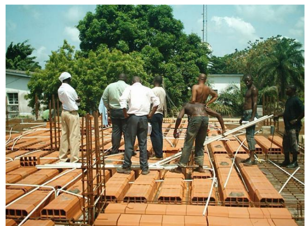
Plate 1: Showing placing of electrical pipes along the clay pots
