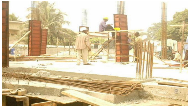
Plate 2: Showing placement of form work for columns
