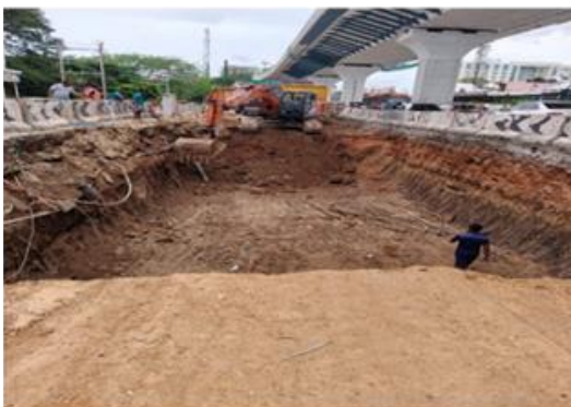
Figure 3.1: Depth of Earth Work Excavation
