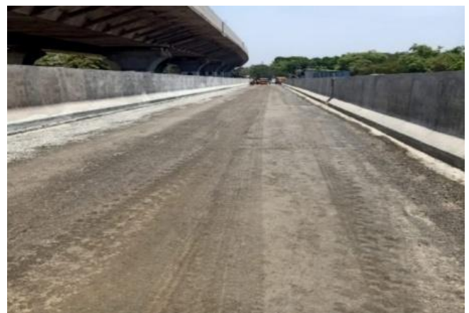
Figure 3.10: Wet Mix Macadam
