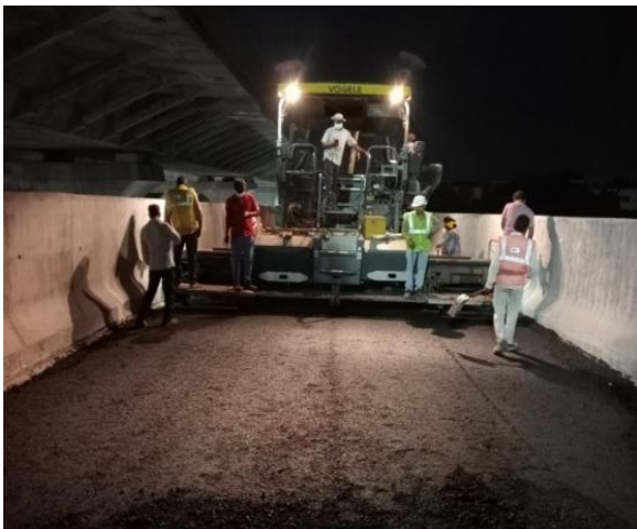
Figure 3.11: Dense bituminous macadam
