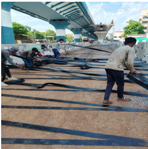
Figure 3.4: Laying of para web
